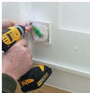
1. Screw the Squebble base plate unit in the correct dwelling location next to active kit with a working power socket within 1 metre (make a note of where the cable exit needs to be).
