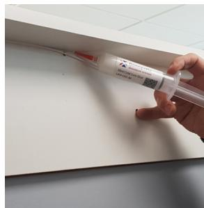
10. Using the Cold Cure Glue, run a bead of glue along the skirting board/wall and push the cable into the glue, keeping tension on the cable for a good finish. Soft tape can be used to hold the cable into the glue until fully cured.
